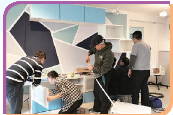
Renovation of Small Group Home by enthusiastic volunteers
