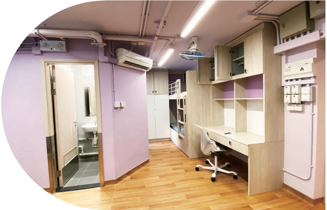
馬可紀念之家的大維修工程竣工，改善宿舍居住環境 The major renovation work of Mark Memorial Home was completed to improve its living environment
