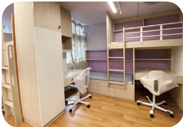
馬可紀念之家進行的大維修工程竣工 The major renovation work of Mark Memorial Home was completed
